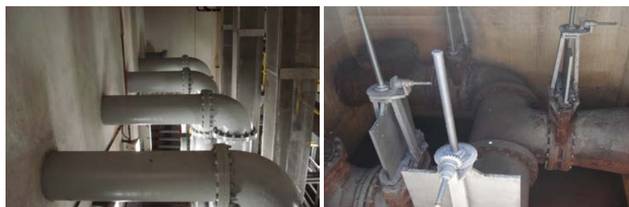
(a) Pump Station at OCSD
