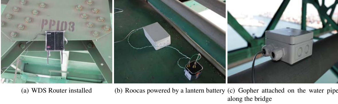
Figure 14. Metal structures of Vincent Thomas Bridge
