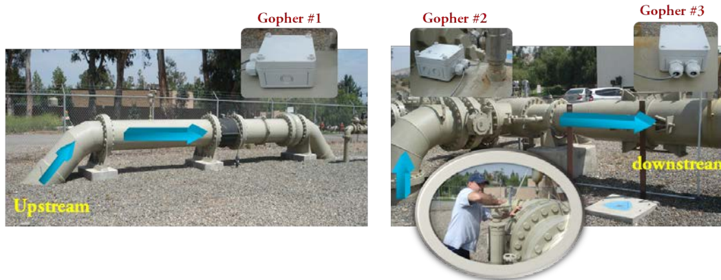
Figure 4. Experimental Setup Showing IRWD Metal Water Pipe
