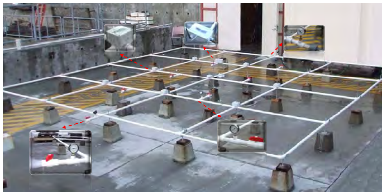
(a) Photo of a 5 \times 5 Water Pipe Network
