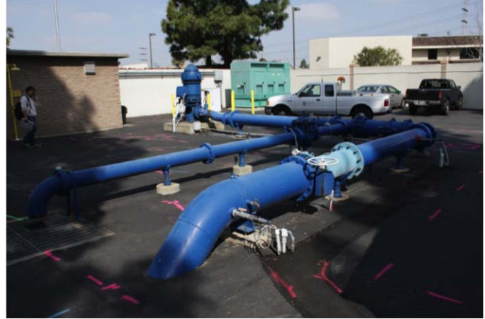
Fig. 11. Experimental Setup Showing PACE Metal Water Pipe
