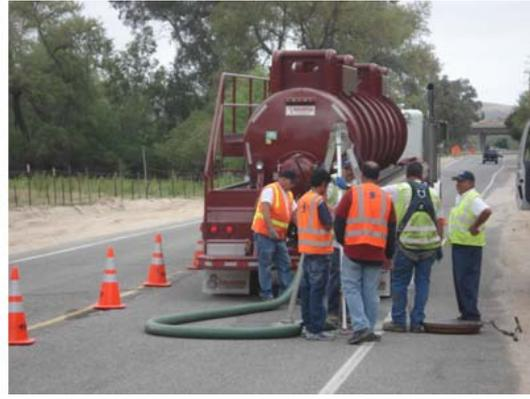
Figure 3. Blowoff hose connection and water tank truck
