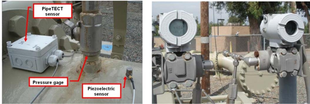
Figure 8. Sensor installation and pressure gages
