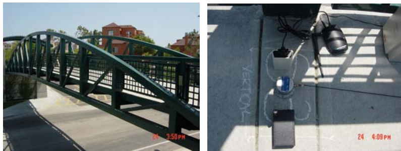
Fig. 8 The Pedestrian Bridge
