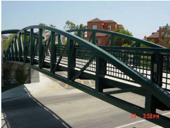
Figure 5. UCI steel truss pedestrian bridge tested with wireless MEMS sensors
